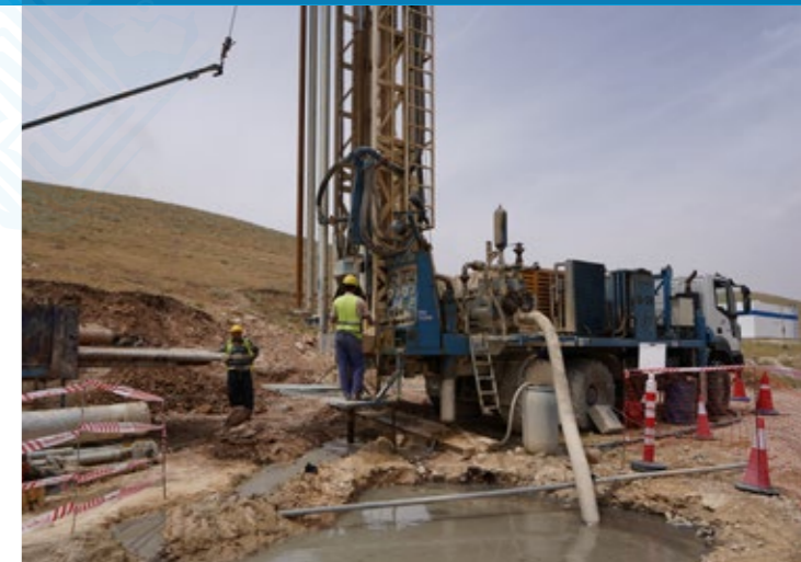
Rehabilitating water facilities. ©UNOPS
