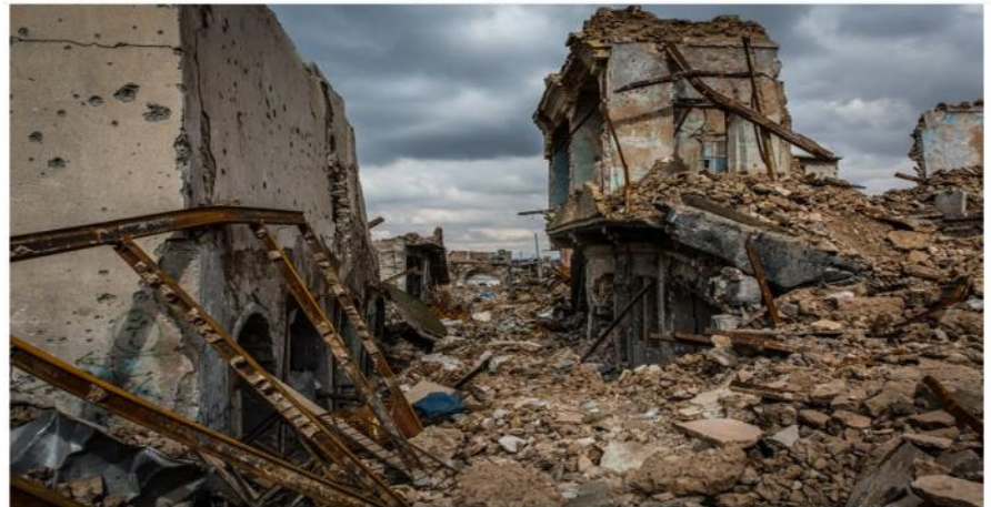
The heavily destroyed Old City district of Mosul, where ISIS militants were cornered, is still littered with unexploded ordnance. Ivor Prickett for The New York Times
