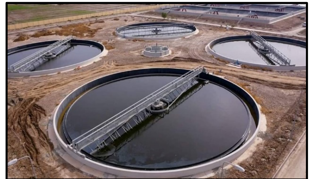
The precipitation Basins-Al-Hai Central Sewage Treatment Plant© Al-Hai District Sewers Directorate
