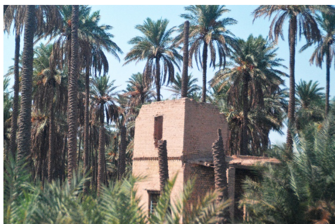
Destroyed property in Muqtadiyah District, Diyala [Photo Credit: OCHA]
