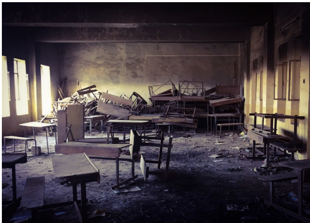
Destroyed school in Sulaiman Baig sub-district, Salah Al-Din Governorate. [Credit: OCHA Kirkuk Sub-Office]
