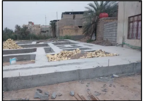
Construction suspended due to high prices - courtesy local contractor
