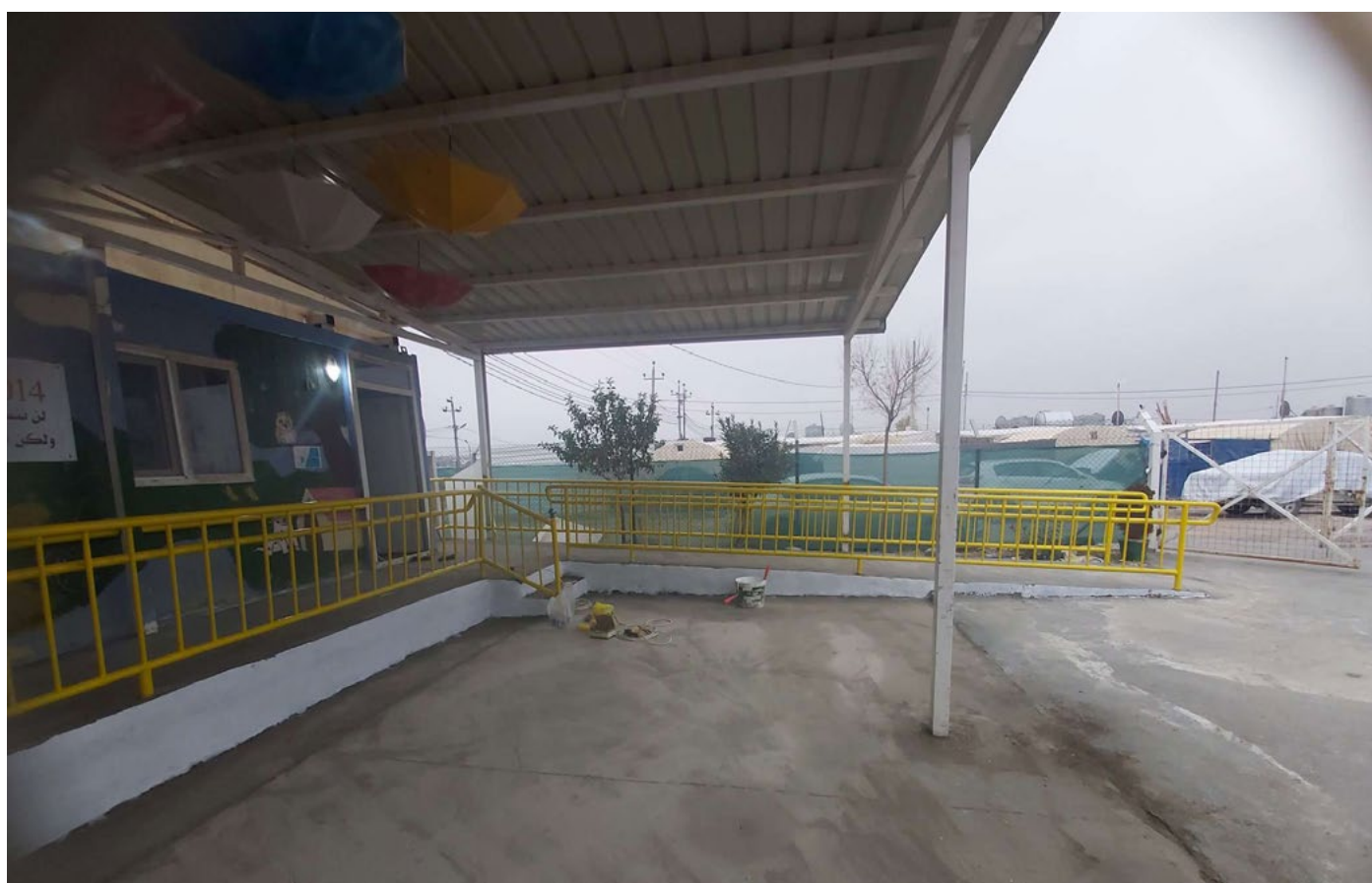
Figure 2: Accessibility works on IOM Community Centre in Dohuk Governorate © IOM Iraq
